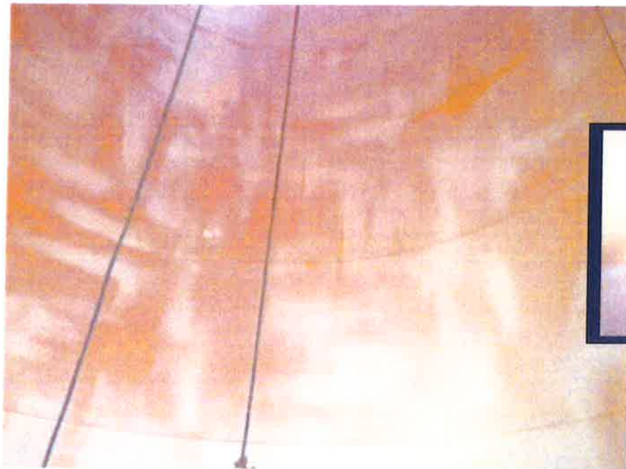
Image #2. May 3. There is a white haze on much of the surface below the normal fill line.
