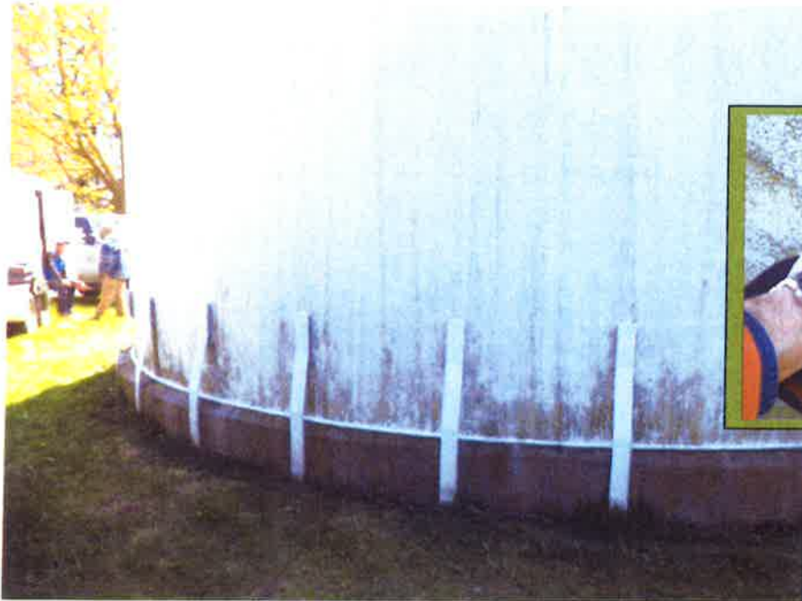
Image #17. May 5th. Mildew visible along bottom of vessel exterior. In some areas, the mold is very thick and well anchored to the surface.
