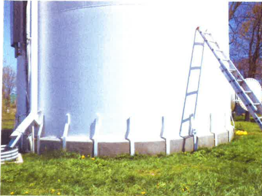
Image #19. May 6th. Cleaned area of the bottom ring.
