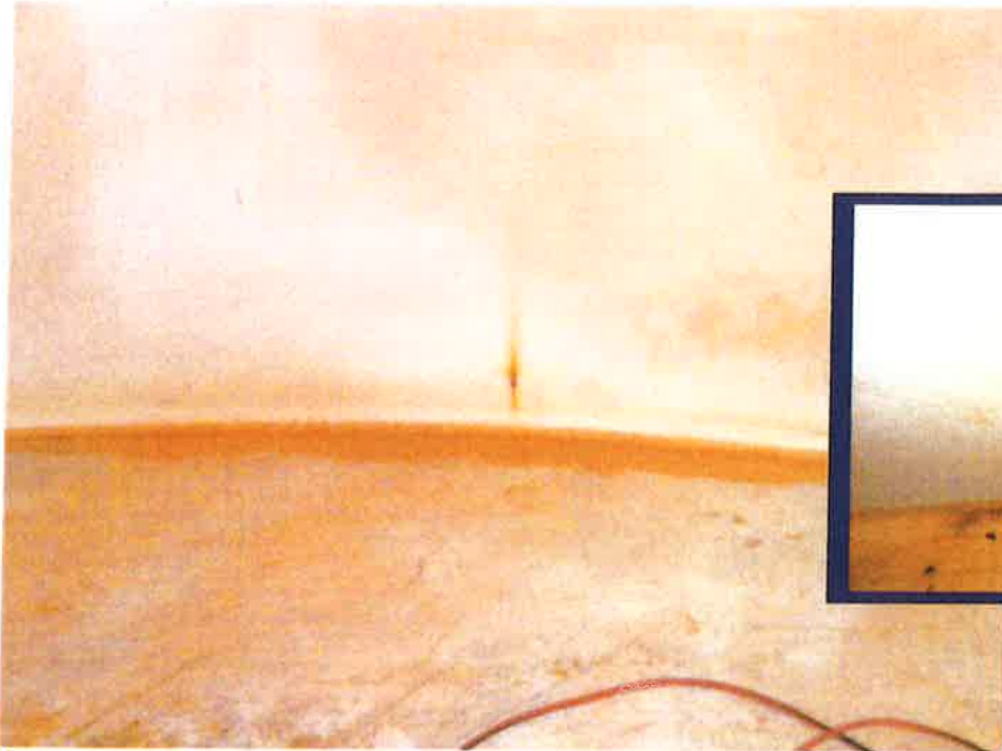
Image #5. May 3. There are a number of small corrosion sites visible.
